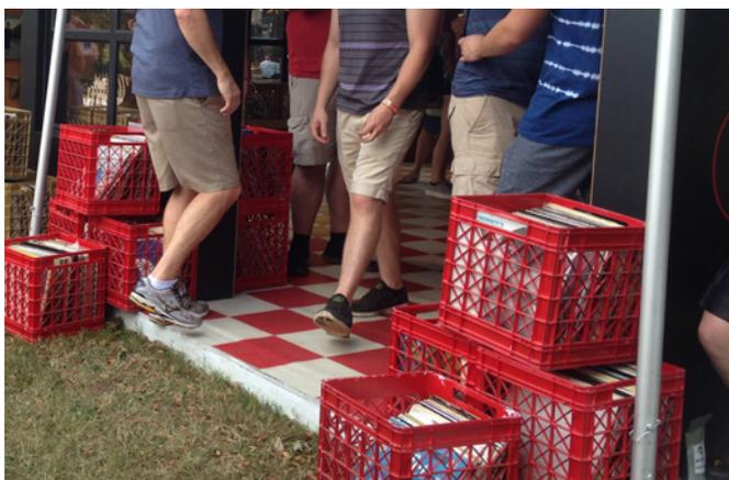
*The flooring leading to the booths is several inches too high and needs ramping to make it accessible. The counter is significantly higher than the 36" maximum.*
