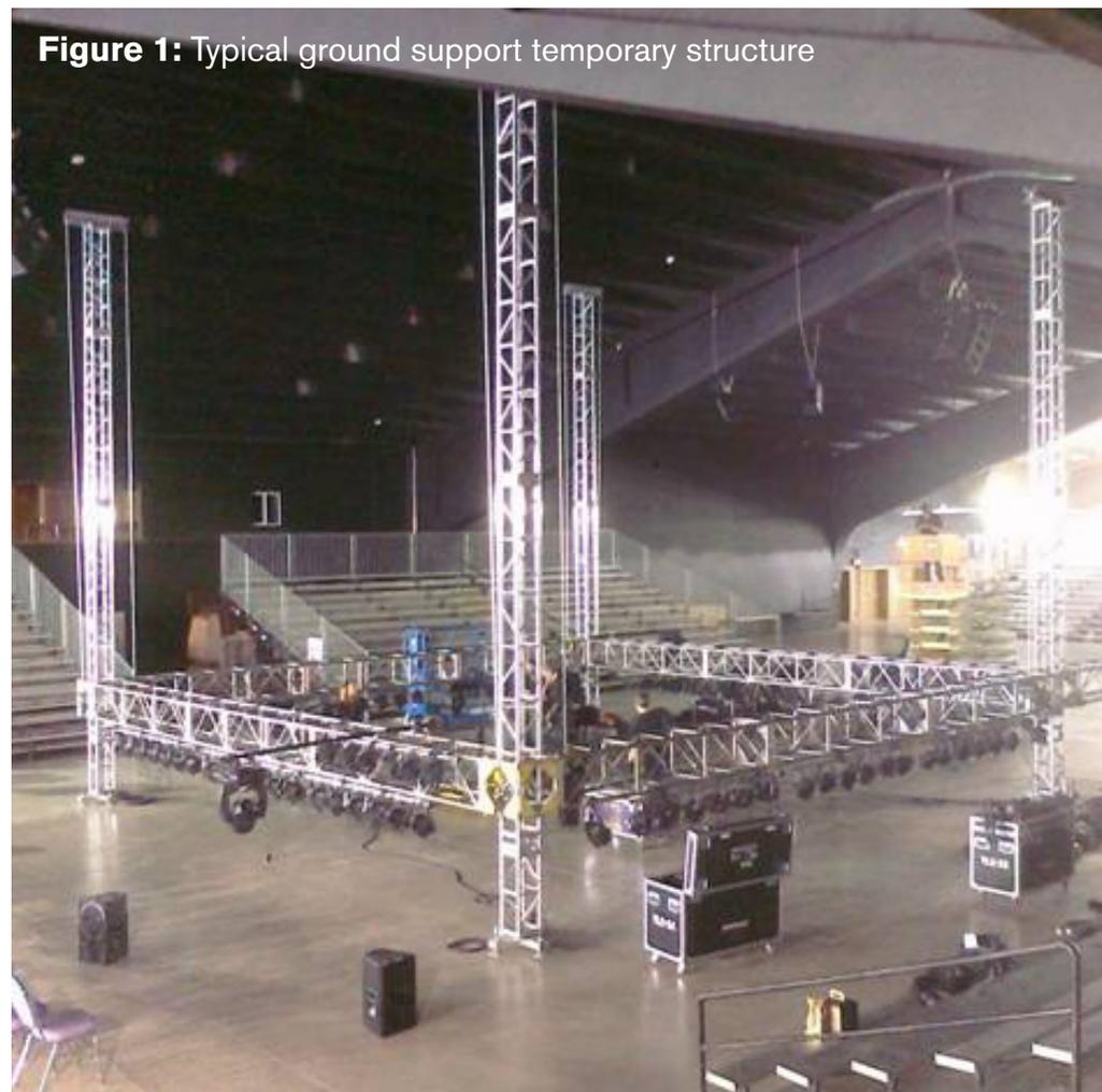
Figure 1: Typical ground support temporary structure
